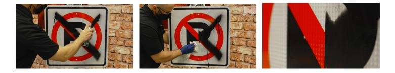
Avery Dennison OL-1000 is a premium clear overlay film ideal for protecting traffic signs. Not only can vandalized traffic signs be cleaned, but when printed with a TrafficJet Print System printer, it will also carry the industry's longest-warranty.
